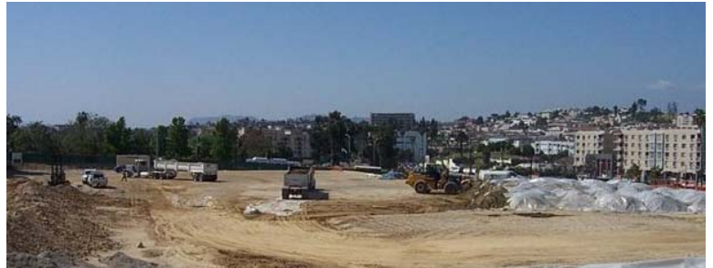
Under Construction - February 2005
